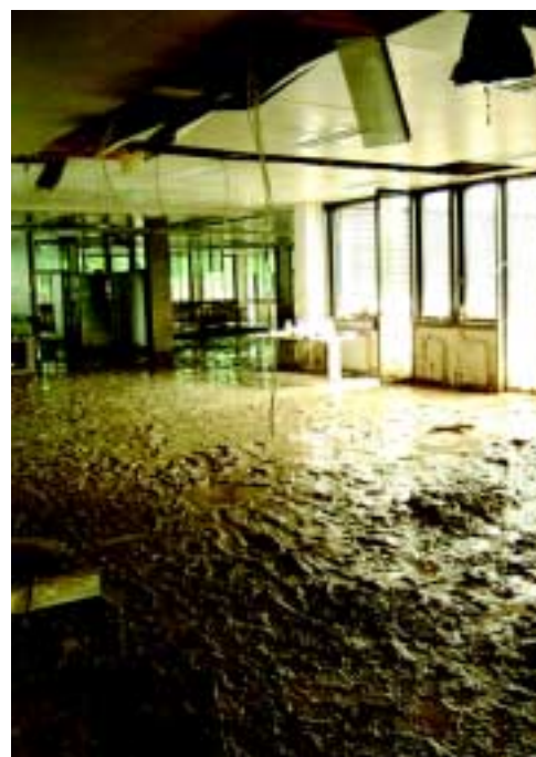
Just one example of the devastation caused by the flood in the office building: water and mud completely destroyed the infrastructure, especially the underfloor EDP network (left); repair and restoration work began with the removal of the old composition flooring. – Right: Things have been back to normal in the purchasing department since the middle of February.
