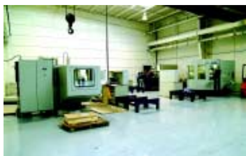
... the new production lines could be installed at the beginning of the new year.
