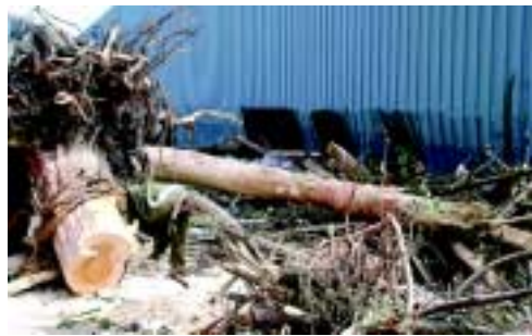
Just one example of many: The machining shop after the flood, from the outside...
